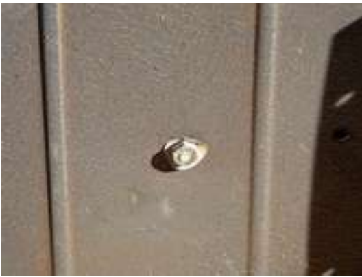
The vertical clamp mounts with a screw that includes a spring washer.
