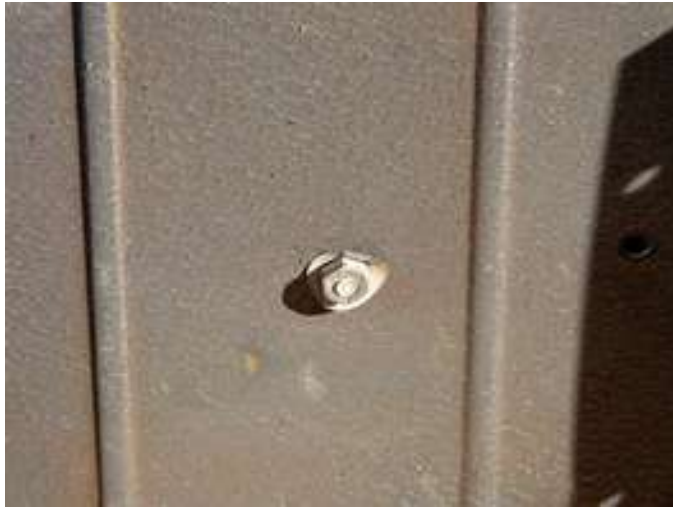
The vertical clamp mounts with a screw that includes a spring washer.
