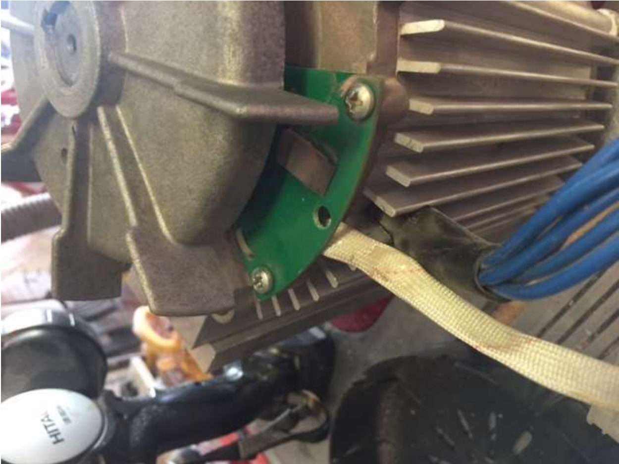
Existing Speed Sensor Under the Fan
